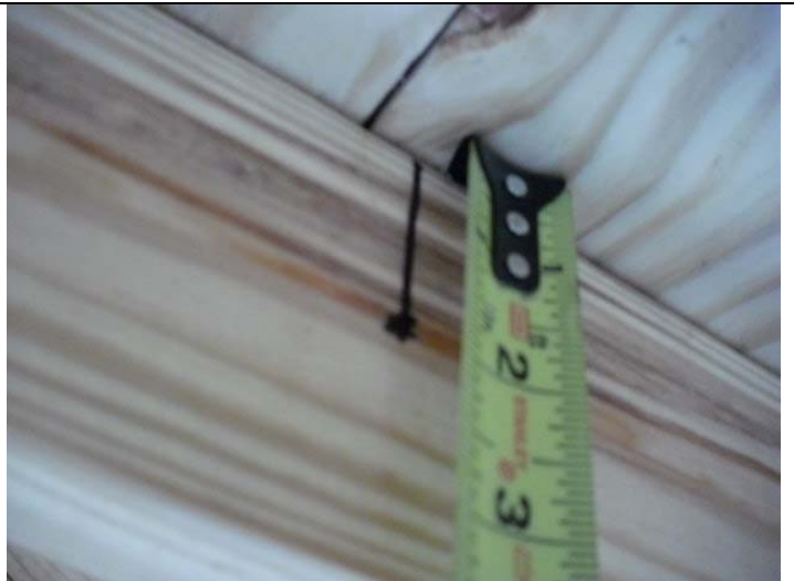
Roof deck attachment
