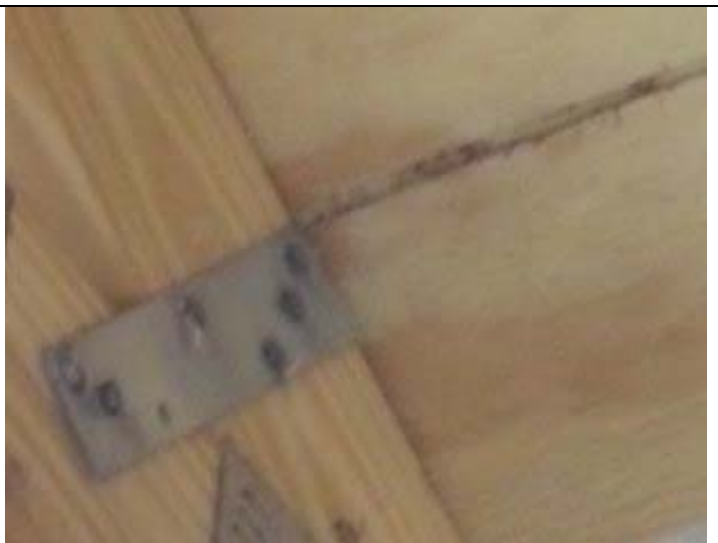
Roof to wall attachment
