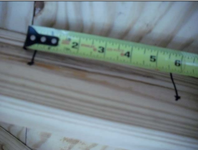
Roof deck attachment
